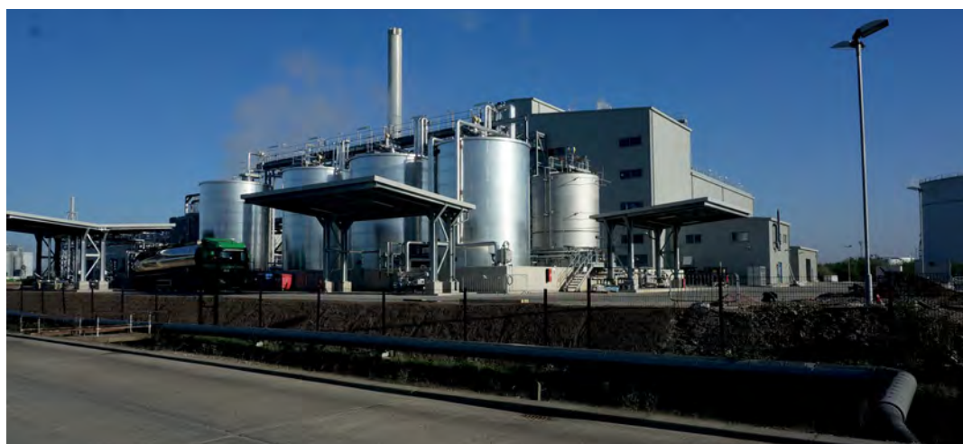
Argent's biodiesel plant
