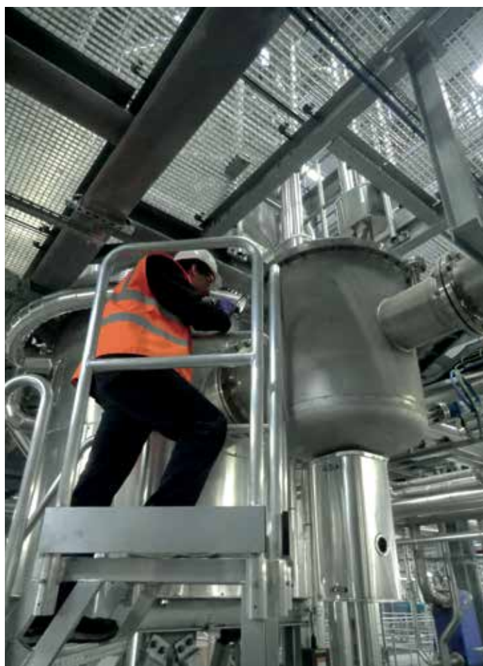
Plant inspection being carried out. Credit: BDI-BioEnergy International
